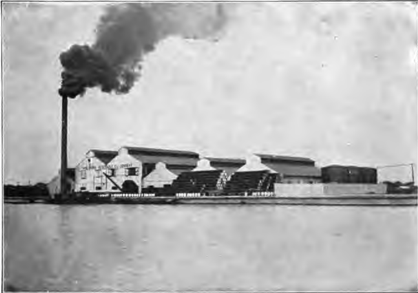
WORKS OF THE PHILIPPINE VEGETABLE OIL COMPANY, MANILA.
